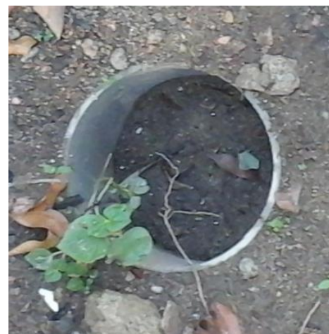
Gambar 5. Lubang biopori
