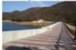
Type4. Parapet wall
